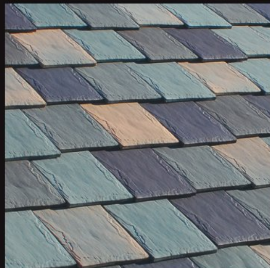
Staggered Installation with Nominal 10" Width
