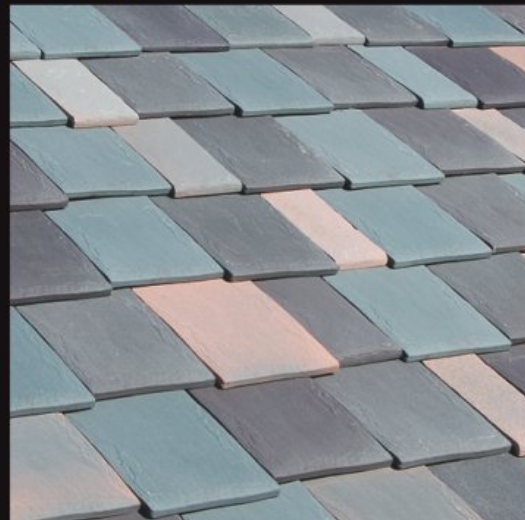
Staggered Installation with Nominal 10", 7" & 5" Widths
